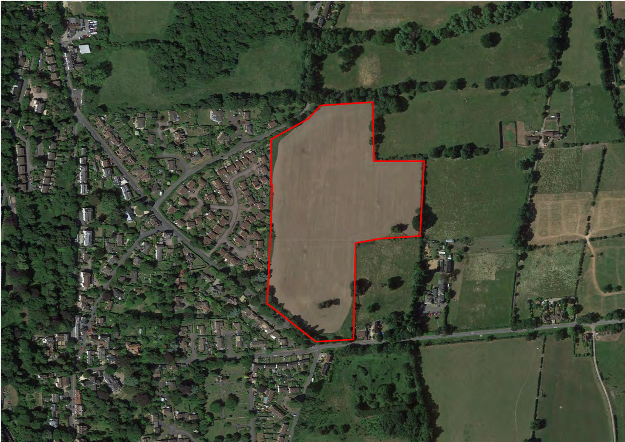
Figure 1: Site Aerial, Red line Boundary
